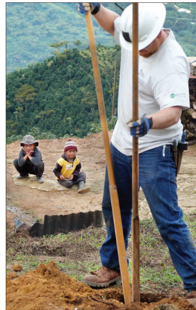
Above: Two Guatemalan men look on as poles are set and then climbed by linemen to install the hardware and, ultimately, string the power lines. Instead of the leg spikes used by Indiana crews to climb the poles, the local lineworkers climb using ropes, knotted into stirrups, which are tied around the poles.
