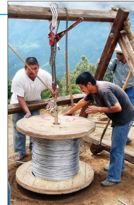
Above: Using a hand chain-hoist, utility pole crossarms and other lumber, the line crews rigged a makeshift frame to support a 1,000-pound "payout reel" of wire allowing it to unroll. Locals keep the coil steady and rolling as the wire is pulled from strand to strand.
